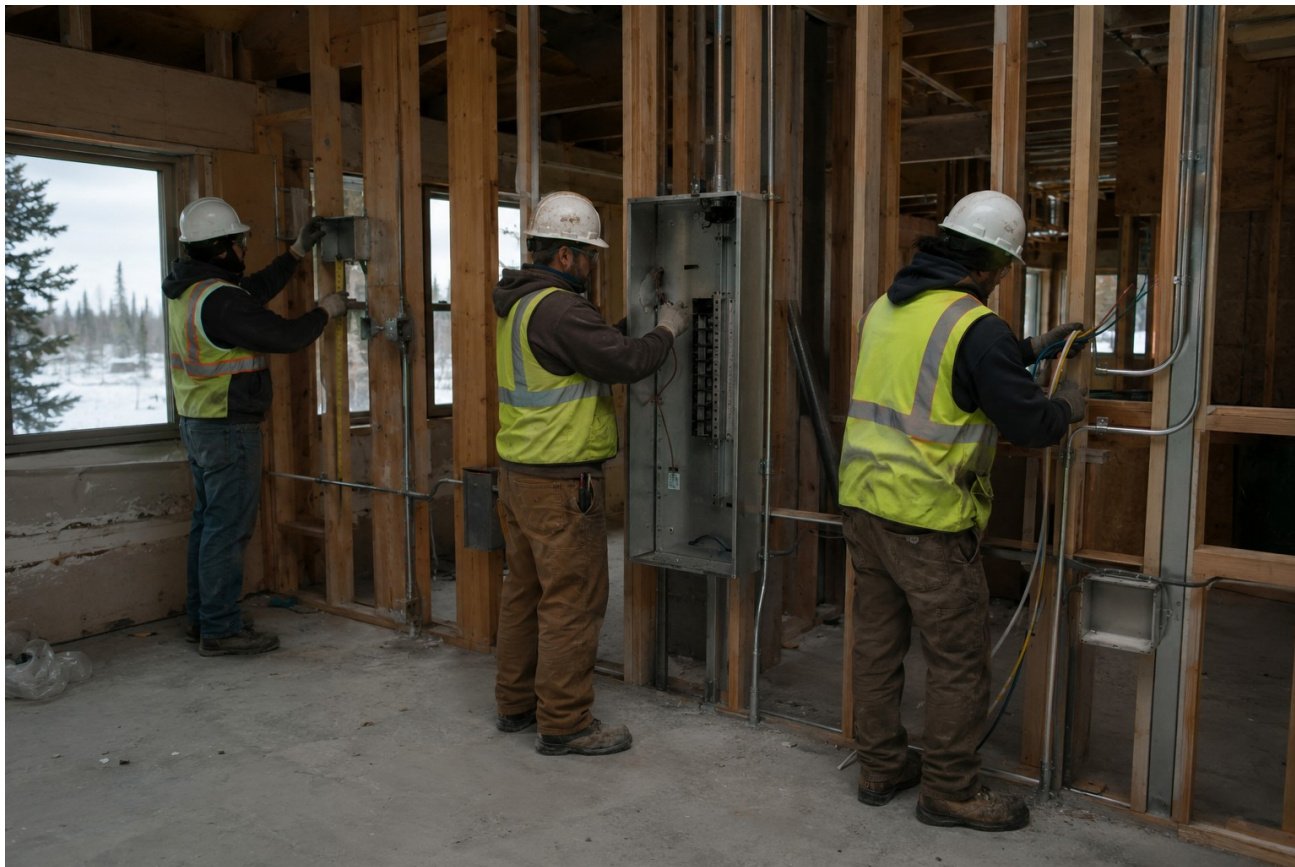
K05-02 - 8 SEP 2027 / 1340: Panel Room 214. Three visible members of the same four-person crew are mounting electrical boxes and panel components and making de-energized terminations; the daily report records all four workers on site. Camera: Government inspection tablet; file hash recorded in report 27-081.
