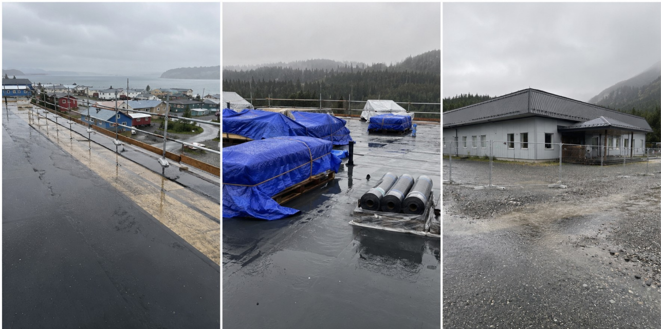
Left to right: partially stripped roof with standing water; secured roofing materials on a wet work surface; Community Support Center exterior during a roofing pause.
